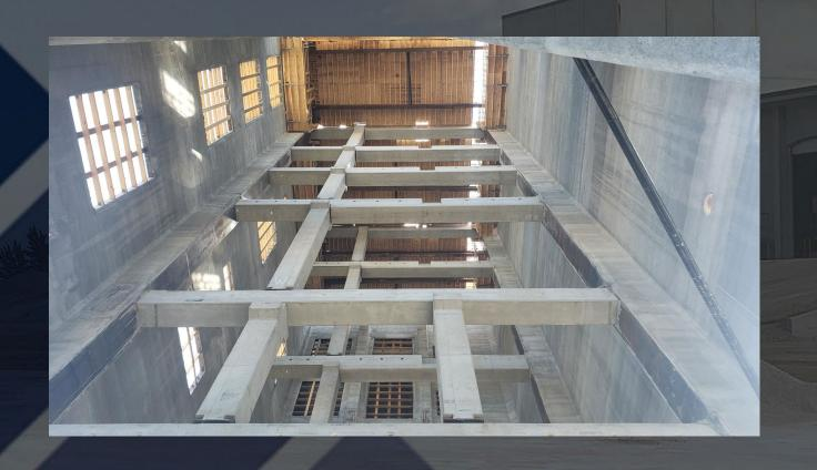
Taracon Precast's precast concrete beams and columns provide the perfect foundation for mounting precast architectural and structural panels, as well as hollowcore slabs. Once erected, the beam and column components offer a seamless and streamlined appearance to the entire structure of the building. We custom manufacture:
