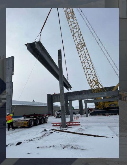
Taracon Precast's double tees are the ideal solution for construction projects that require strength, beauty, and flexibility within large structures with high load capacities for floor and roofing systems. Double tees are usually manufactured in a range of standard widths and spans.
